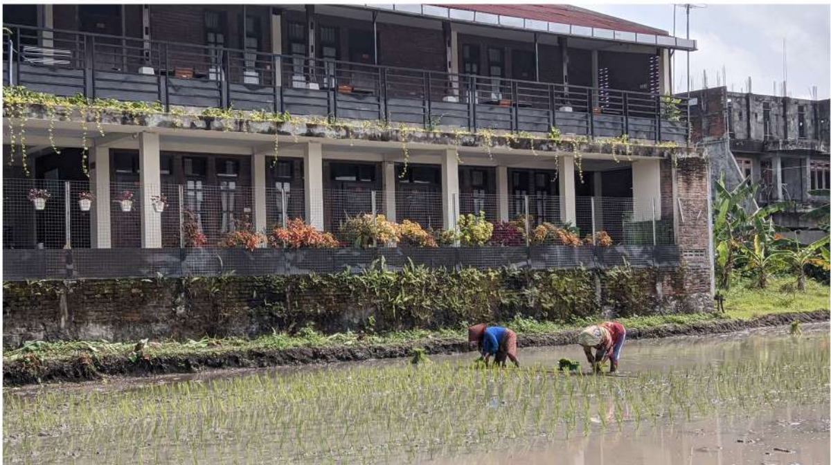
Kompleks Griya Jagadhaya (1) Griya Jagadhaya Complex (1)
